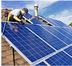
How People Are Paying Next to Nothing for Roof Solar...
